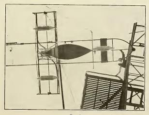
${\bf Fig.~3}$  Hoisting aerodrome to Launching-track
